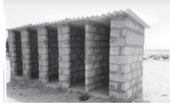
Temporary toilets put up by PSDF-Alliance for tsunami victims
